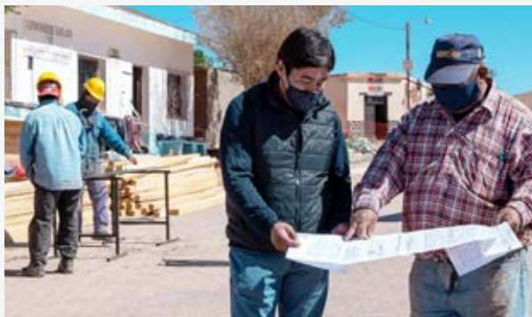
▼ Expansion and remodeling of the Tolar Grande Health Center
