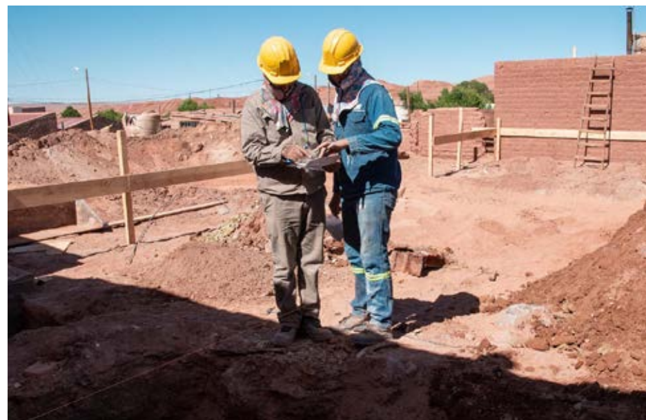
▲ Lindero health centre construction team
