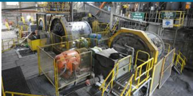
Photo: Caylloma Mine- 1,250 tpd processing plant
