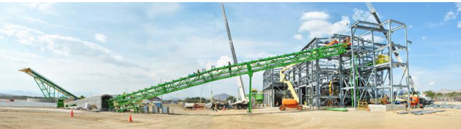
Photo: San Jose Mine- Processing plant ore transport conveyor belt system
