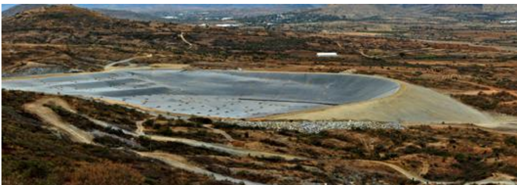
Photo: San Jose Mine- Tailings Dam
